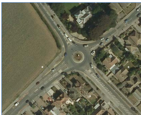
Figure 16 - A256 / A255 Dane Court Roundabout
